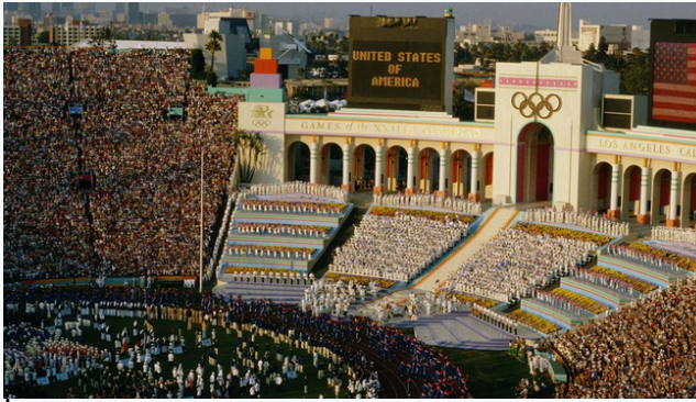
The Los Angeles '84 Olympic Stadium
